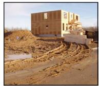
Rain could easily wash this loose soil into the storm sewer and into a nearby stream, causing a water quality standards violation that could cost the site operator up to \$37,500 each day it occurs.
