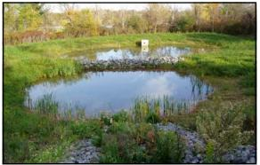
Stormwater retention ponds provide effective water quality control by using forebays for sediment settling, and have controlled-discharge outlets for flood control.
