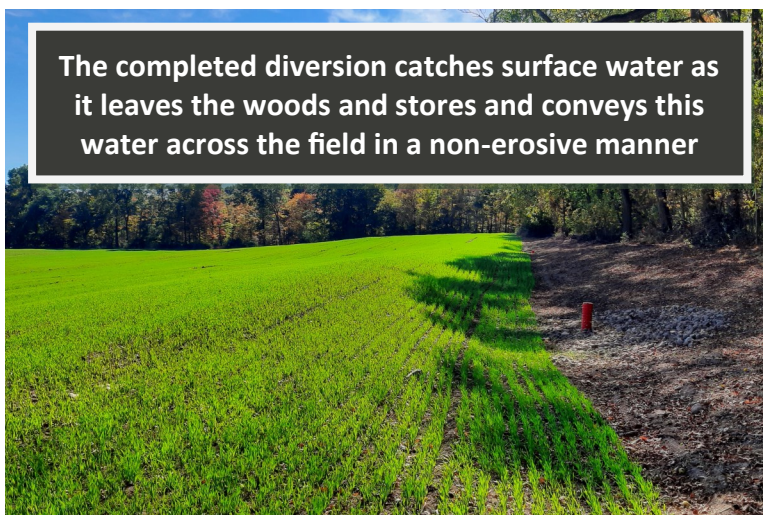
The completed WASCOB after the field was planted to wheat this fall. The subtle design creates 100% farmable short-term water storage while greatly reducing downslope erosion
